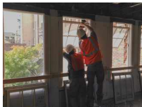
An example of a window re-installation
