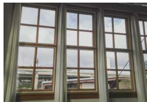
Office windows post-installation
