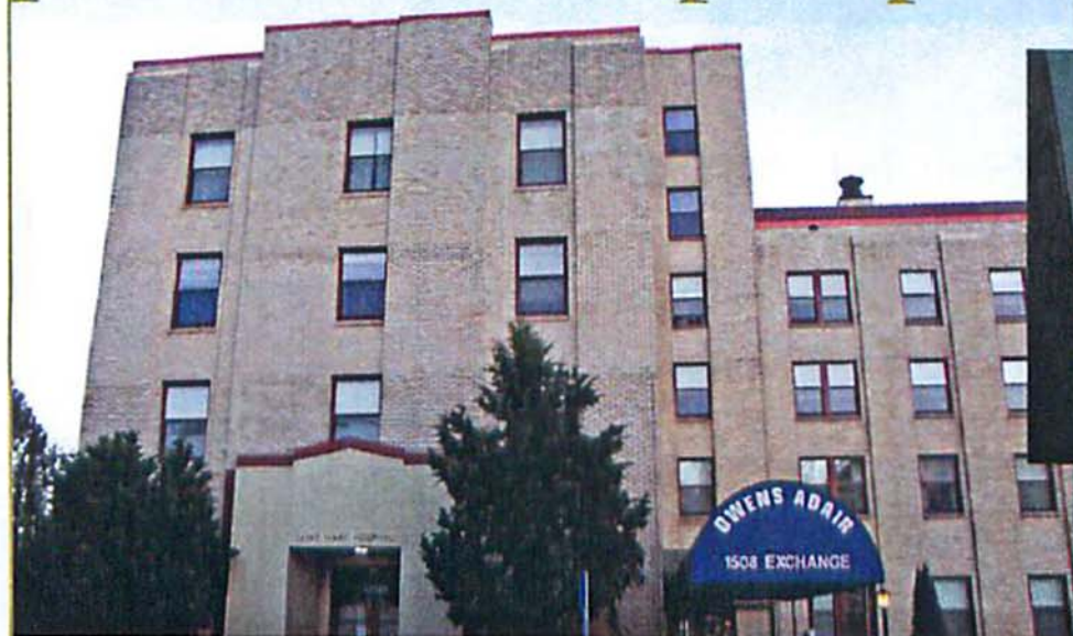
LEFT: The building's windows are now good as new; repairing them proved the most cost-effective option. ABOVE: Pre-work, the windows were showing significant damage.
